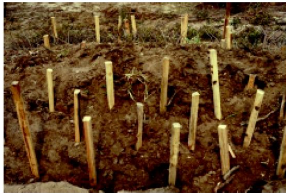
Figure 16-11b Each layer of branches is followed by a layer of compacted soil (Robbin B. Sotir & Associates photo)
