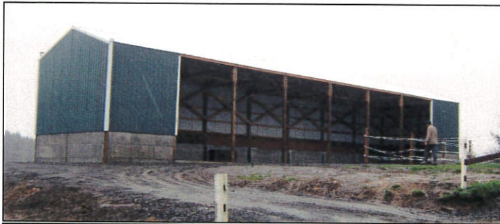
2,300 square foot manure storage facility on a horse ranch near Lincoln City is a result of a project between Lincoln SWCD and landowner. It provides 500 cubic yards storage during rainy months.
