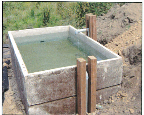
Developed spring provides alternative off-stream water source for livestock on a Siletz Ranch
