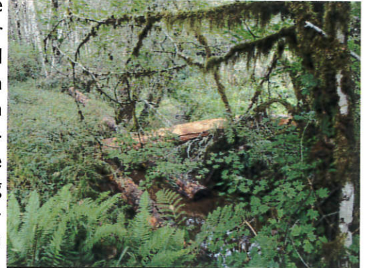
Large wood placed in Flynn Cr (Alsea Watershed) to increase juvenile salmon habitat
