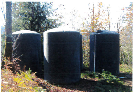
20,000 gallon rain water storage facility near Baker Creek, upper Siletz River
